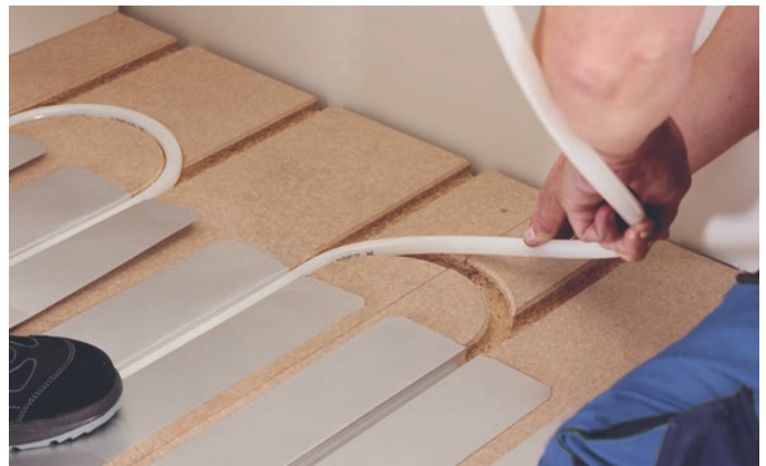
Figure 10 Mounting the heating pipe.
