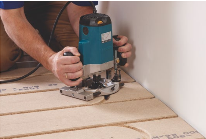
Figure 7 Cutting turning grooves in every 2nd row.
